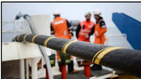
Fig. 4: Installation process of 3x150 mm<sup>2</sup> copper MV XLPE Submarine cable
