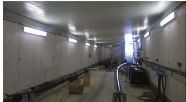
**Fig. 11: 320kV DC premoulded joint installed in tunnel**
