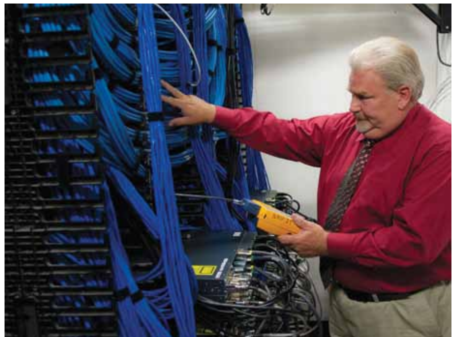
Bob Weber, senior manager of infrastructure services for NKU, is shown here testing a link in one of Griffin Hall's telecommunications rooms.
