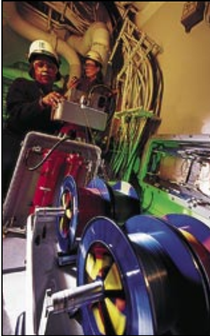
Once the tubes are in place, a two-person crew then uses specialized blowing equipment that delivers clean, compressed air to quickly and easily propel up to 12 optical fibers through each tube.
